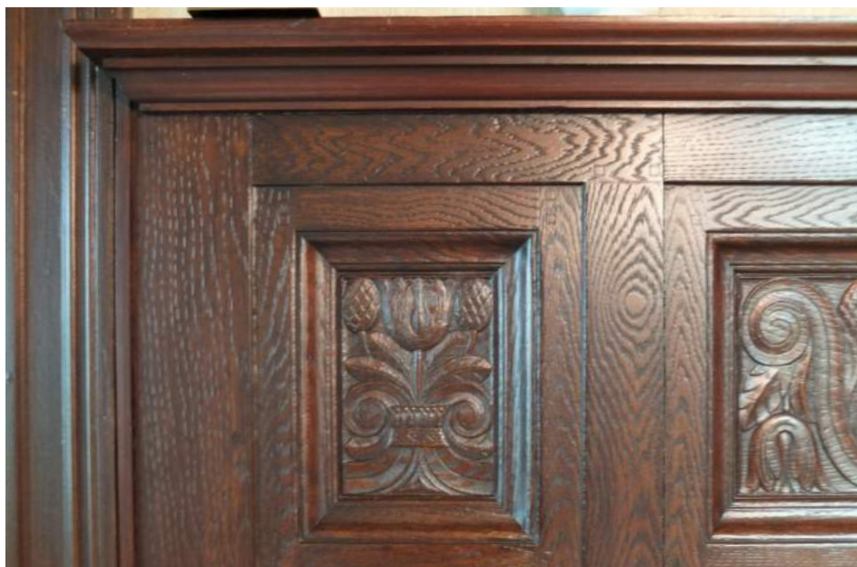
Afb. 51: Details lincrusta-lambrisering
